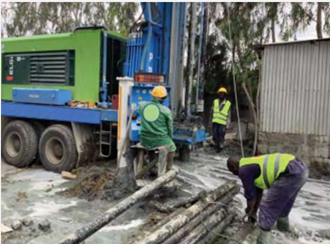
Drilling of bore hole
