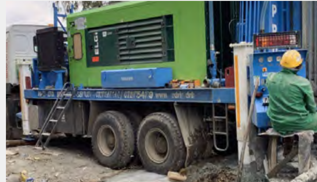
Drilling of borehole
