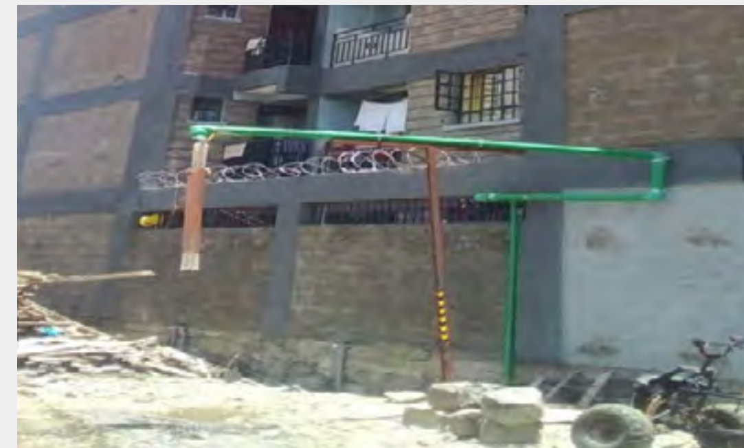
Progress of the borehole to connection to the residence
