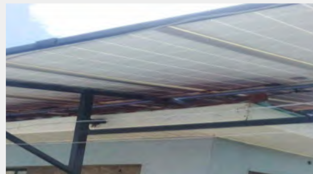
Solar panels installed
