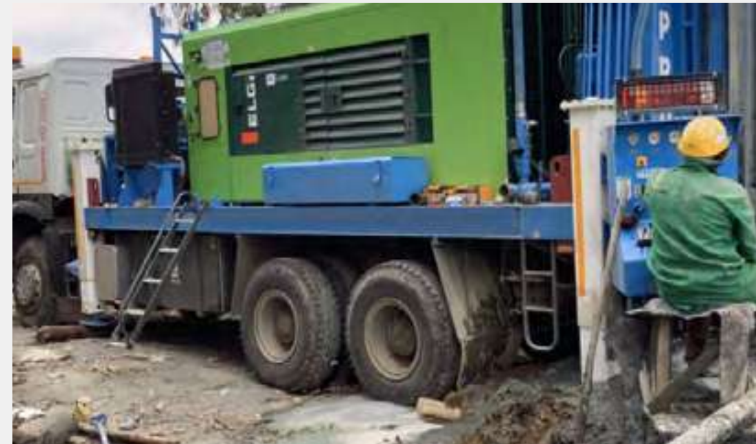
Drilling of borehole
