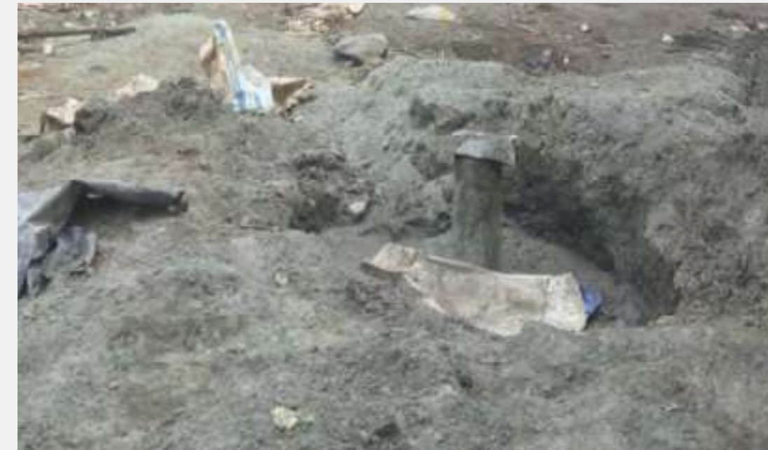
Progress of the borehole to connection to the residence
