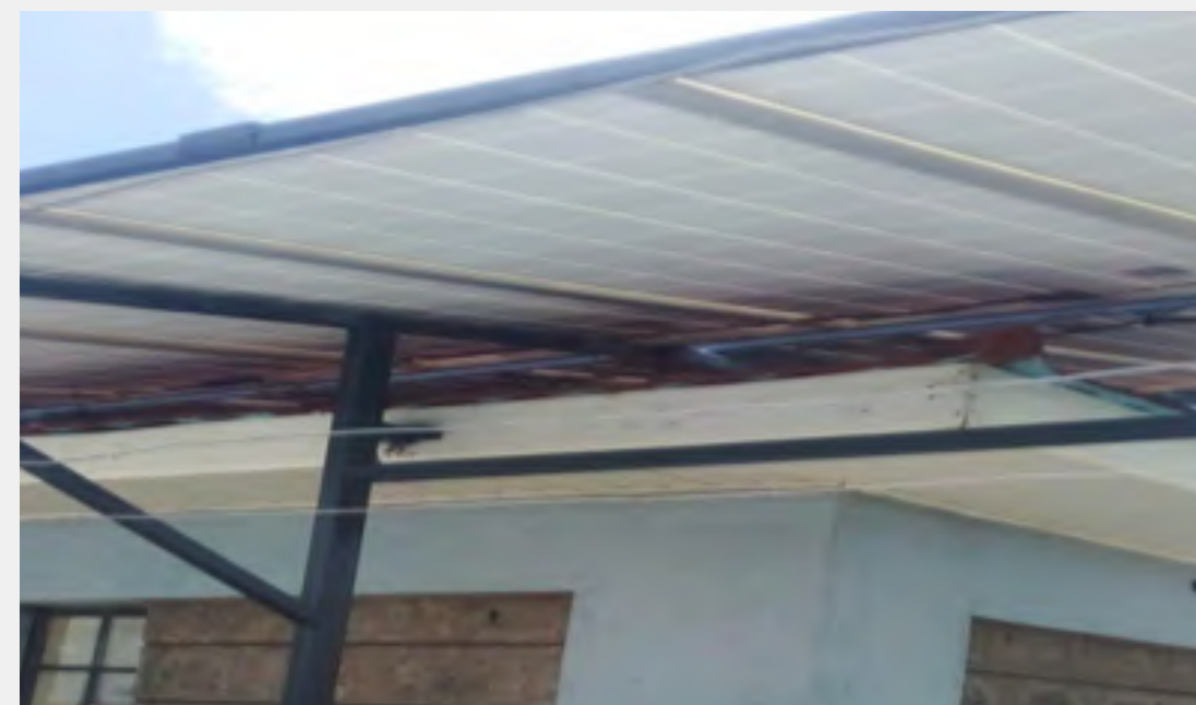
Solar panels installed
